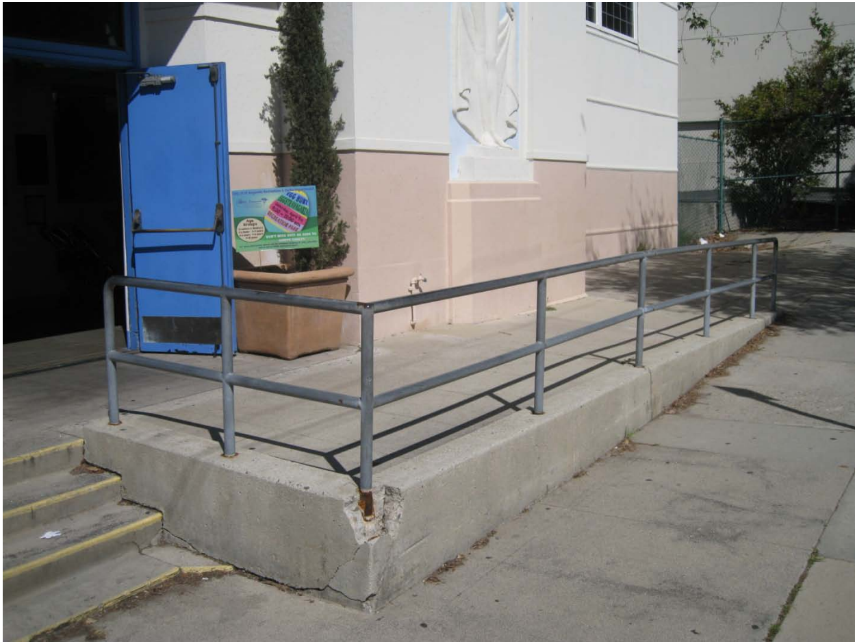
Ramp from Mariposa for wheelchair access.
