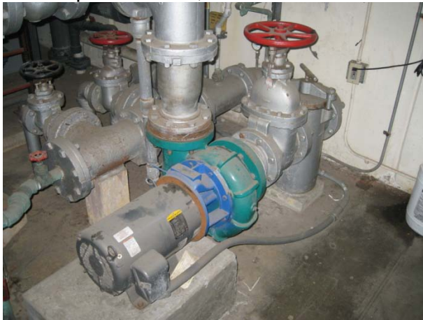
Pool recirculation pump with strainer - picture of below deck pool piping.
