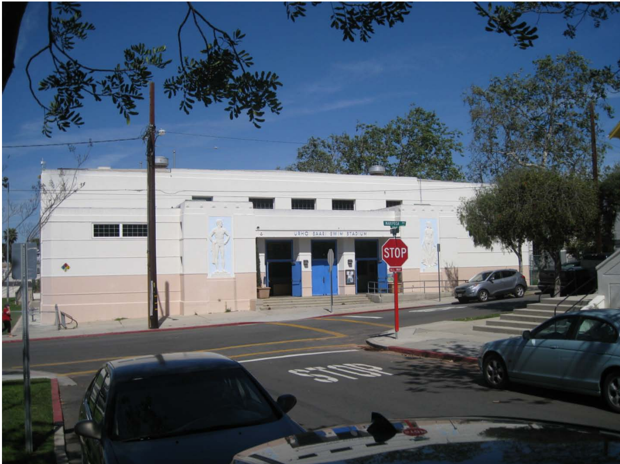
View of swim stadium from frontage along Mariposa Avenue
