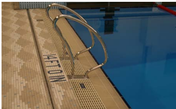
Example of Rim Flow Gutter Also called Flush Deck
