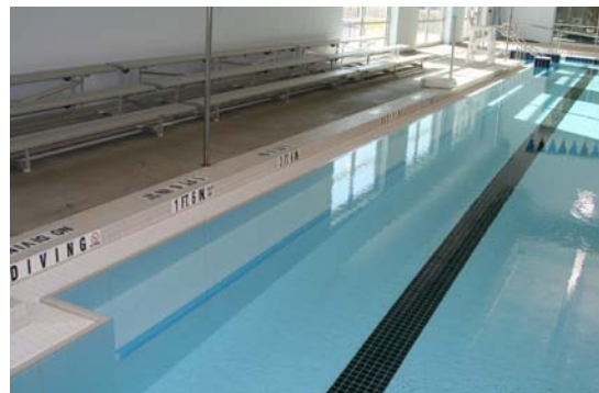
Example of Rim Flow with Riser
