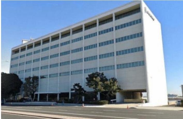
Figure 1 Existing Facade 650 NPCH
