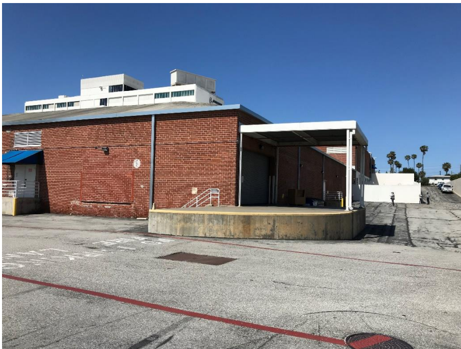
Photograph 7. View of the east and north facades facing east. Taken May 1, 2020.
