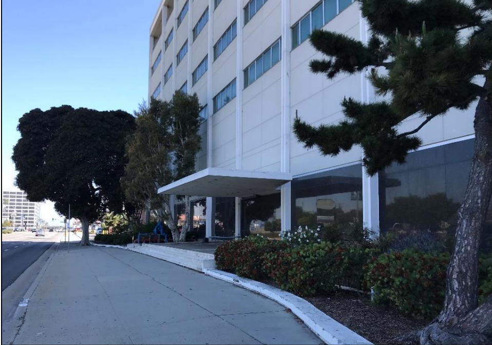
Photograph 6: View of former entrance on the western façade of the building located at 650 North Pacific Coast Highway, facing northeast. Taken May 1, 2020.
