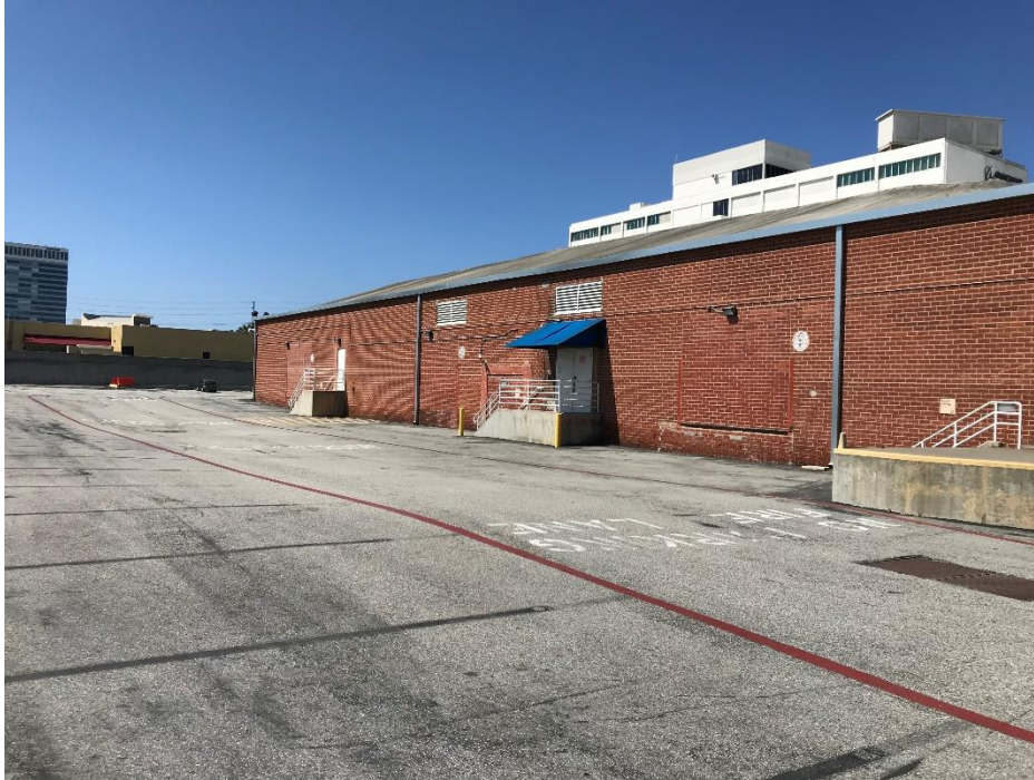
Photograph 8. View of the east façade facing southwest. Taken May 1, 2020.
