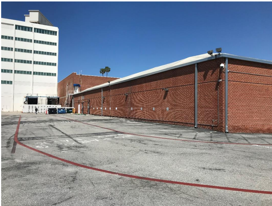
Photograph 9. View of the south façade facing northwest. Taken May 1, 2020.
