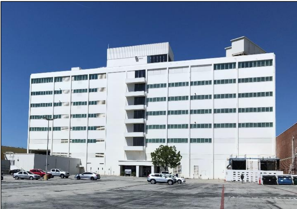
Photograph 7: View of eastern façade of the building located at 650 North Pacific Coast Highway, facing west. Taken May 1, 2020.
