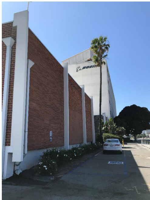
Photograph 5. View of the west façade facing south. Taken May 1, 2020.
