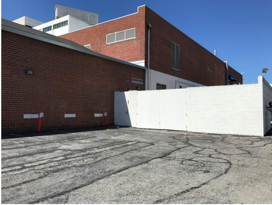
Photograph 6. View of the north façade facing southwest. Taken May 1, 2020.
