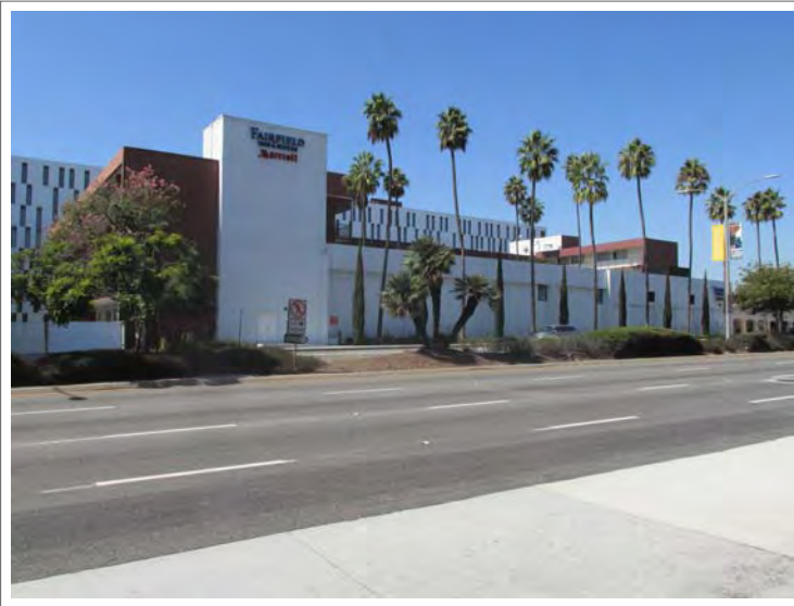
Photo A: Northwest facing view of the Fairfield Inn and Suites Hotel from Pacific Coast Highway
