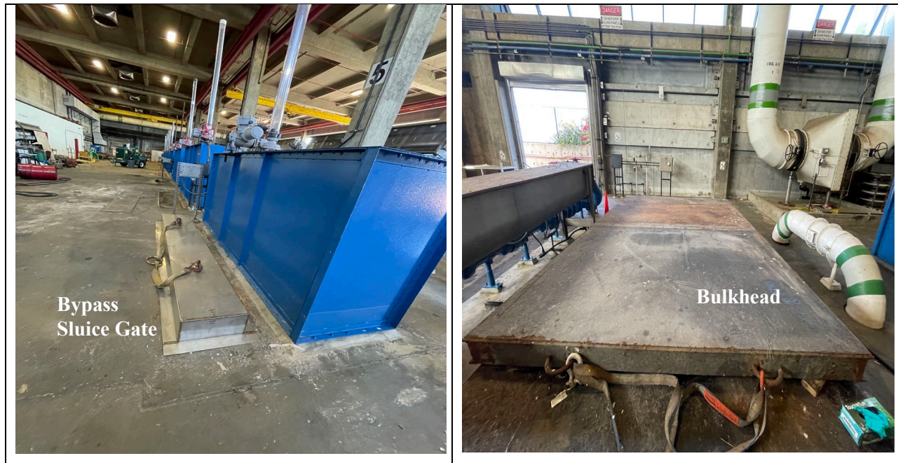
Figure 15 –Bypass Sluice Gate (Left) and Bulkhead (Right)
