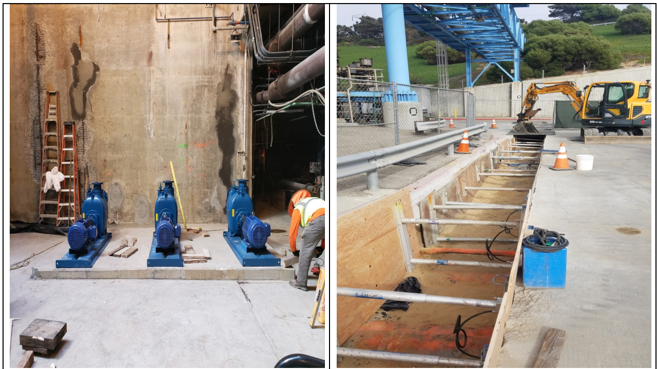
Figure 35 – Central Storm Drain Rerouting Project (in Construction)
