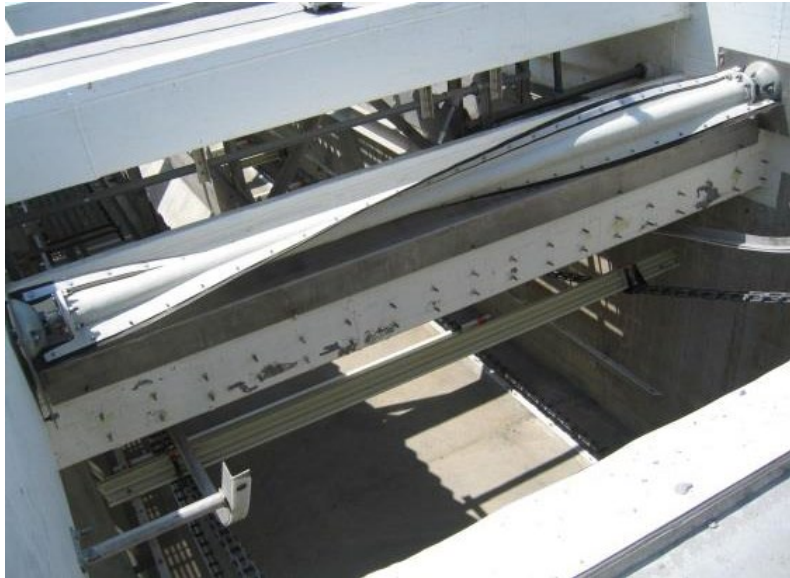
Figure 6 – Primary Tank Skimmers
