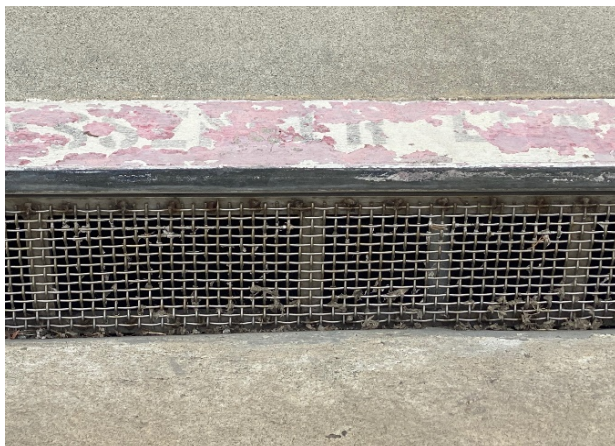
Figure 22 – Screen and Grill on Catch Basin
