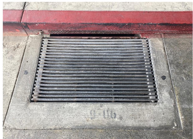
Figure 22 – Screen and Grill on Catch Basin
