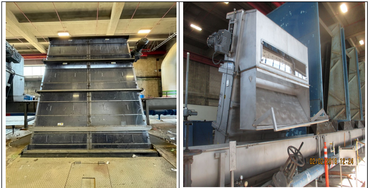
Figure 33 – Headworks Barscreen
