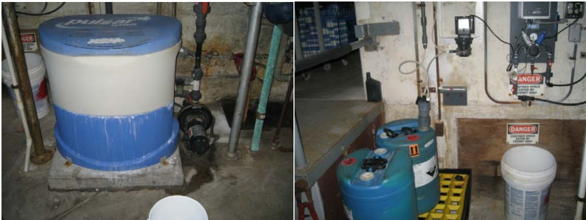
Chlorine erosion feeder and Stenner metering pump for acid to regulate pH – all controlled with automated controller
