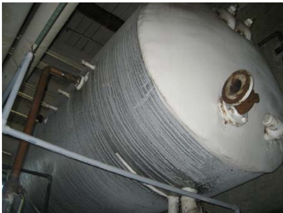
Domestic hot water storage tank for showers, etc. & hot water boiler for domestic supply.
