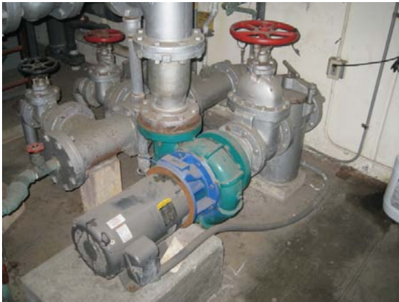
Single recirculation pump for both pools – pump motor is 208-230/460v, 41-38/19A, 1760 RPM, 15HP, 3 ph
