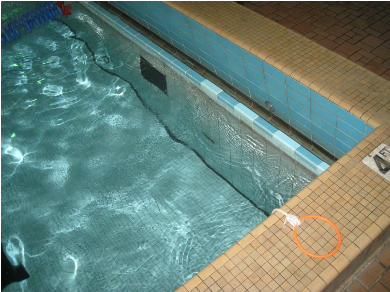
Typical tiles pool vessel and scum gutter – note; water is low by about two inches at time of photograph
