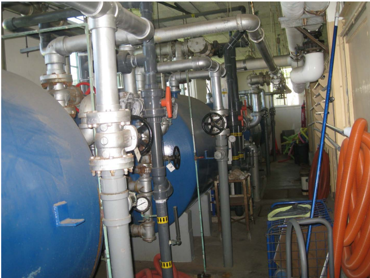
Existing rapid sand filters from original construction with iron pipes, typical of four (4)
