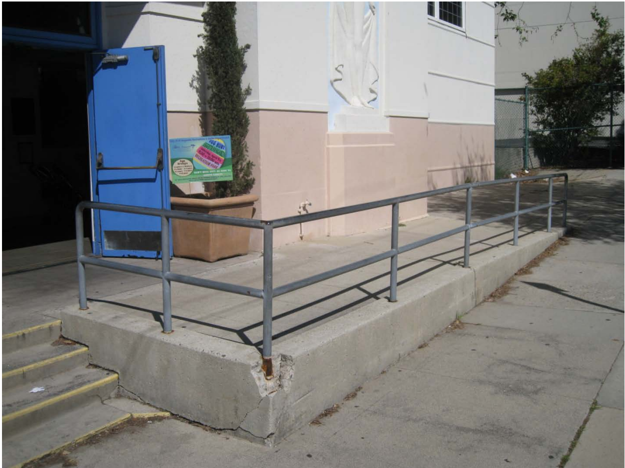
Ramp from Mariposa for wheelchair access.
