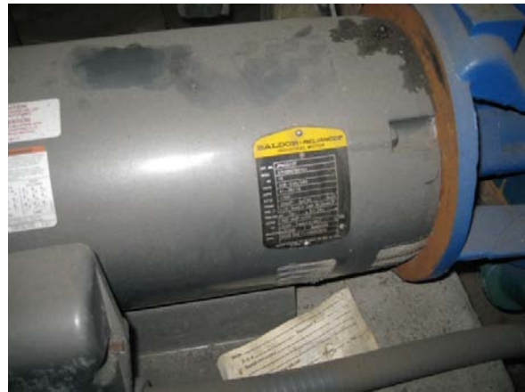
Single recirculation pump for both pools – pump motor is 208-230/460v, 41-38/19A, 1760 RPM, 15HP, 3 ph
