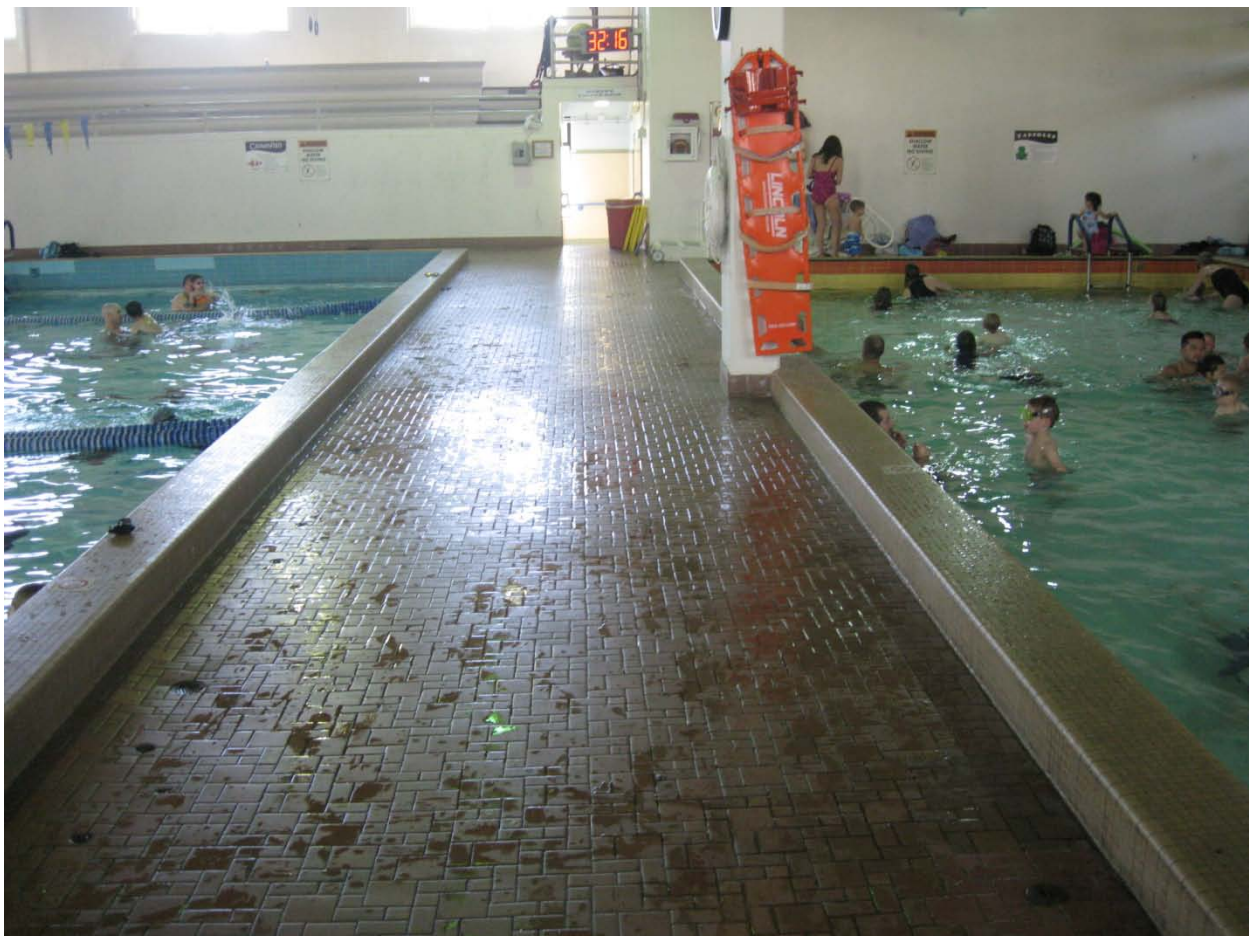
Deck area between pools, note curbs around each pool typically – which defeat ADA accessibility.
