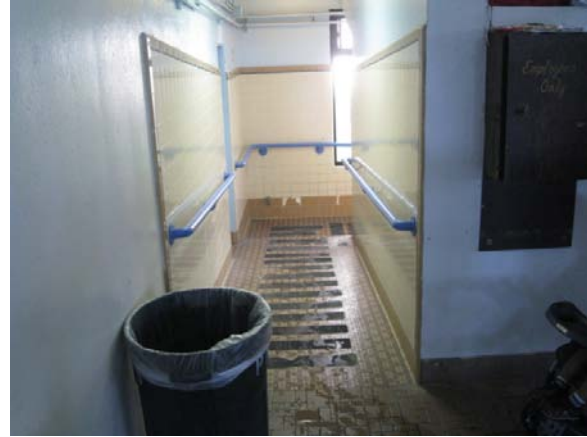
View of ramp access to changing area and from changing area with abandoned Pedilieu and rinse.
