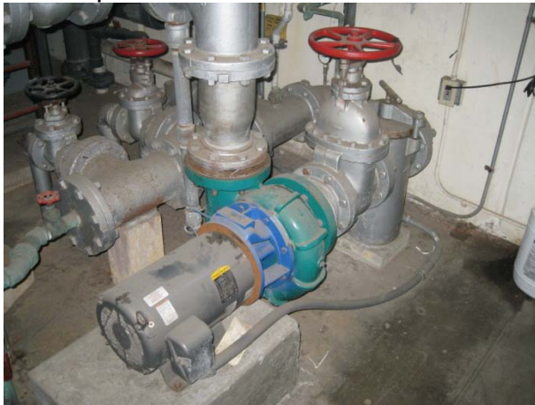
Pool recirculation pump with strainer - picture of below deck piping.
