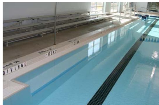
Example of Rim Flow with Riser
