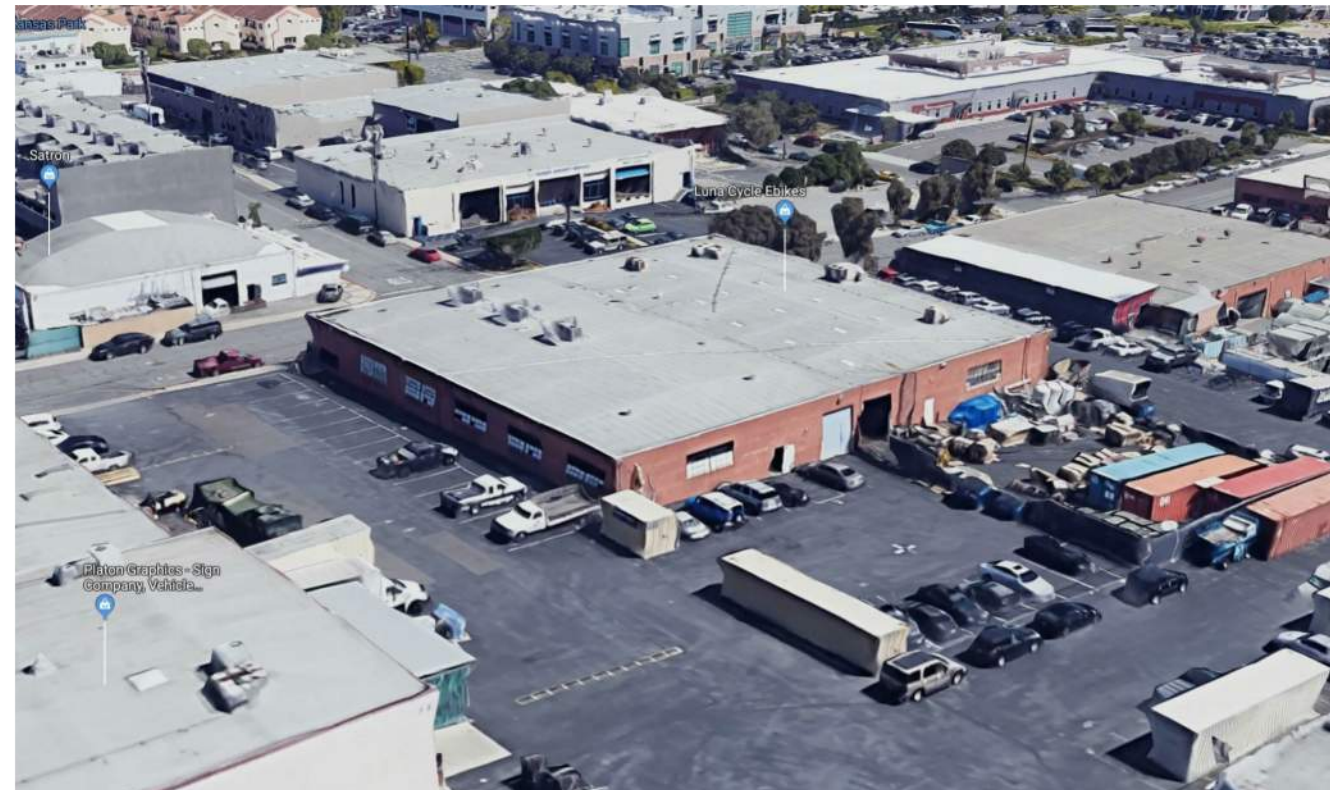
VIEW FROM SOUTHWEST
