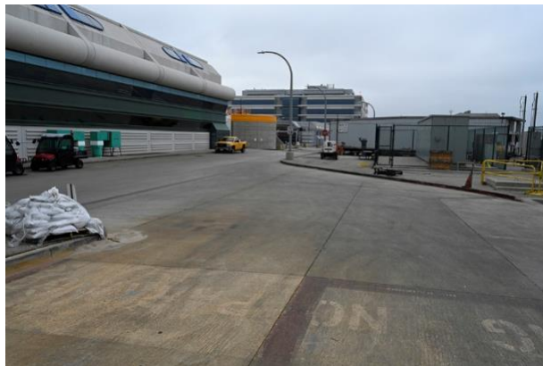
Figure 22: Road and parking area where flood waters flowed to the secondary treatment part of the plant.
