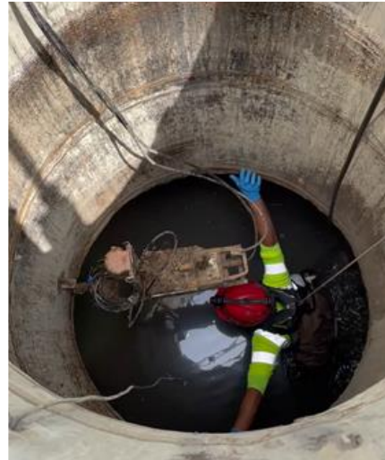
Figures 28 and 29: Left: Sewer Scout™ buoy prior to be deployed into the conveyance system. Right: Confined space entry to a maintenance hole to retrieve the buoy.
