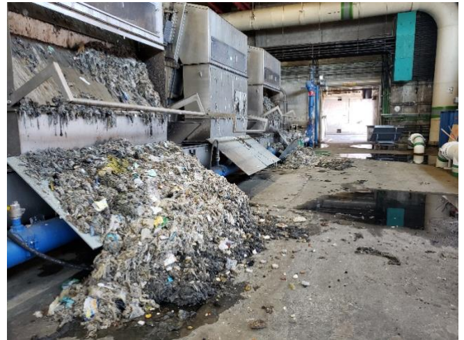
Figures 7 and 8: Back sides of the bar screens, opened to remove screenings (instead of using the sluice).
