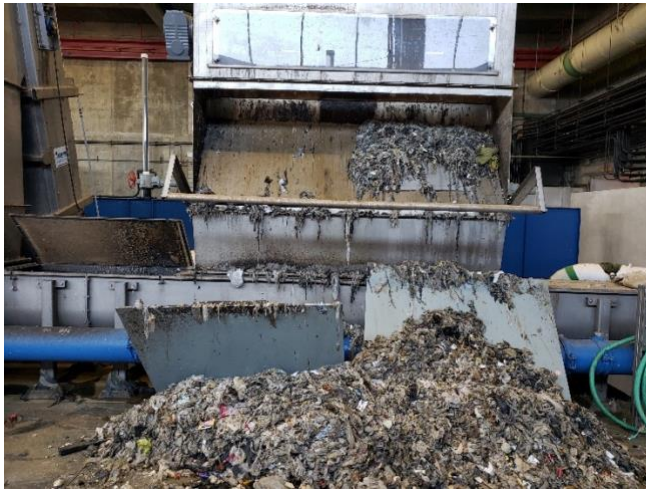
Figures 7 and 8: Back sides of the bar screens, opened to remove screenings (instead of using the sluice).
