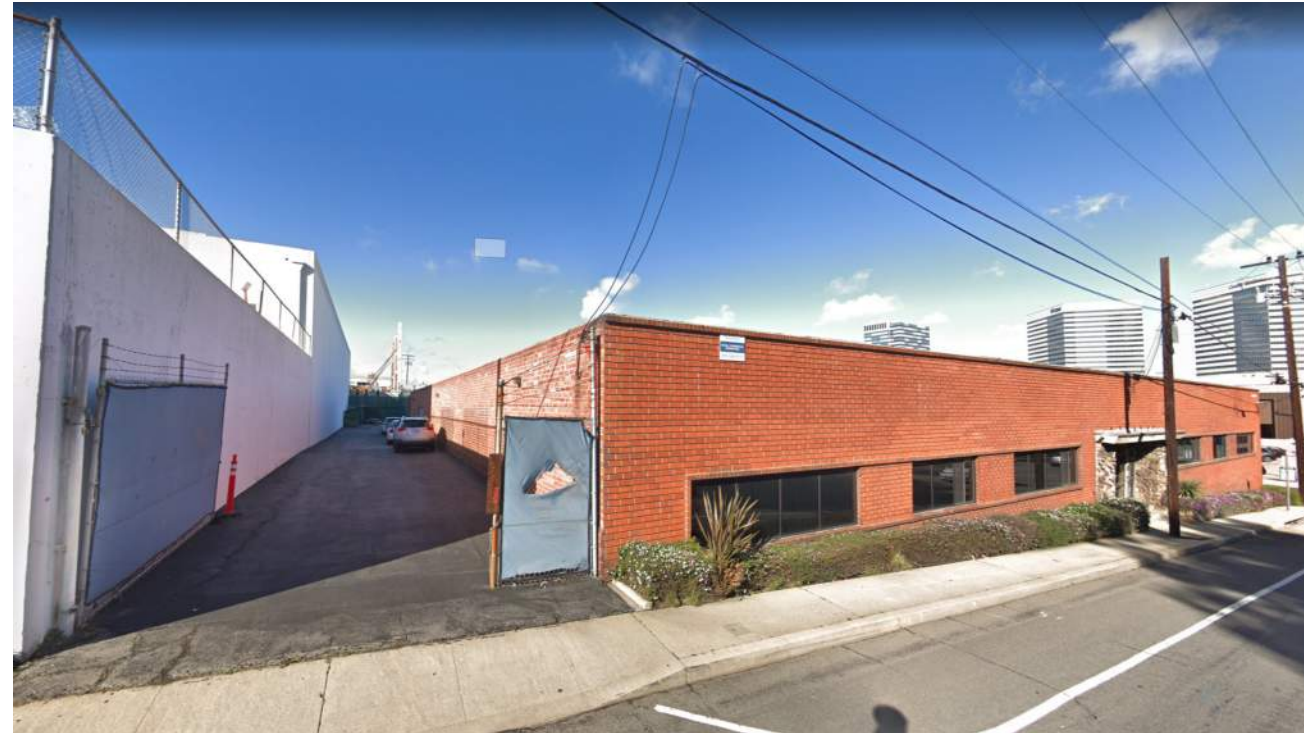
VIEW FROM SOUTHWEST
