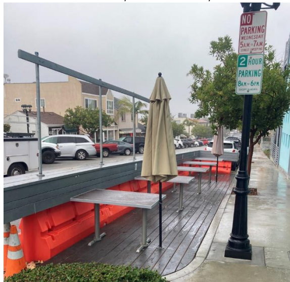
Figure 17 - Parklet on Richmond Street north of Grand Avenue
