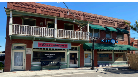
218-220 Richmond Street is one of the few remaining examples of a mixed-use commercial building from the 1910s
