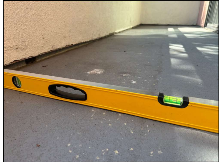
Slope for drainage appears adequate.
