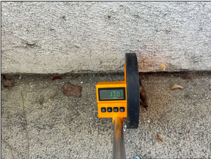
Measurement of balcony in one direction.
