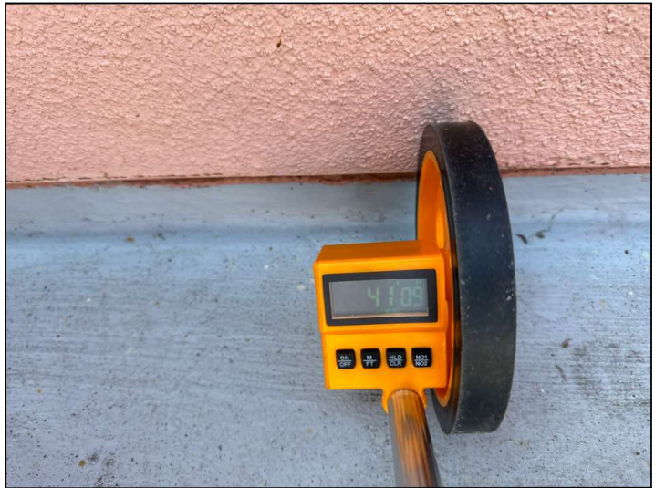
Measurement of balcony in one direction.
