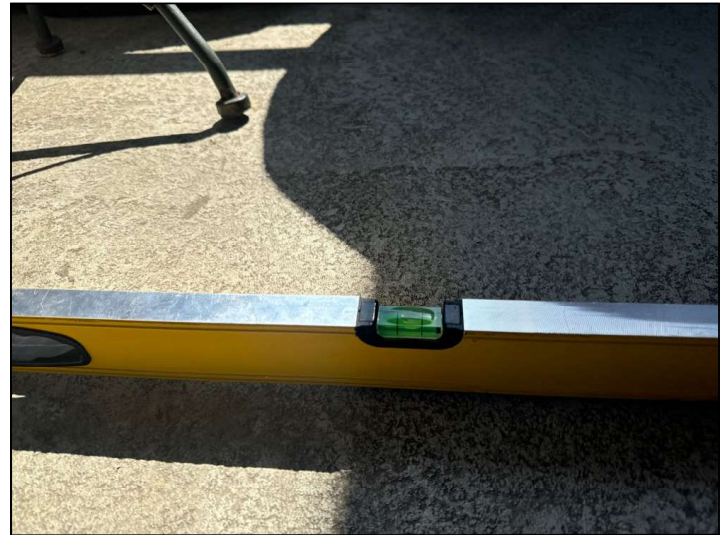
Slope for drainage appears adequate.
