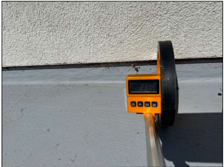
Measurement of balcony in one direction.
