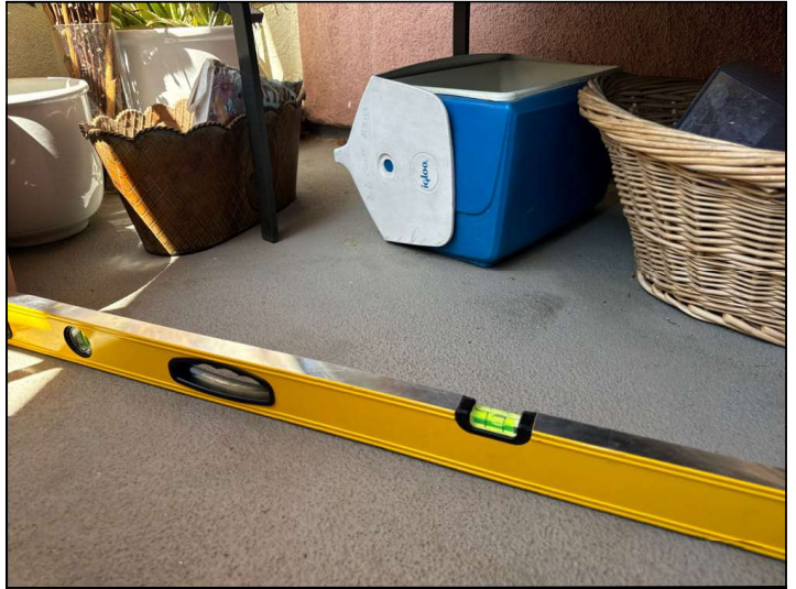
Slope for drainage appears adequate.
