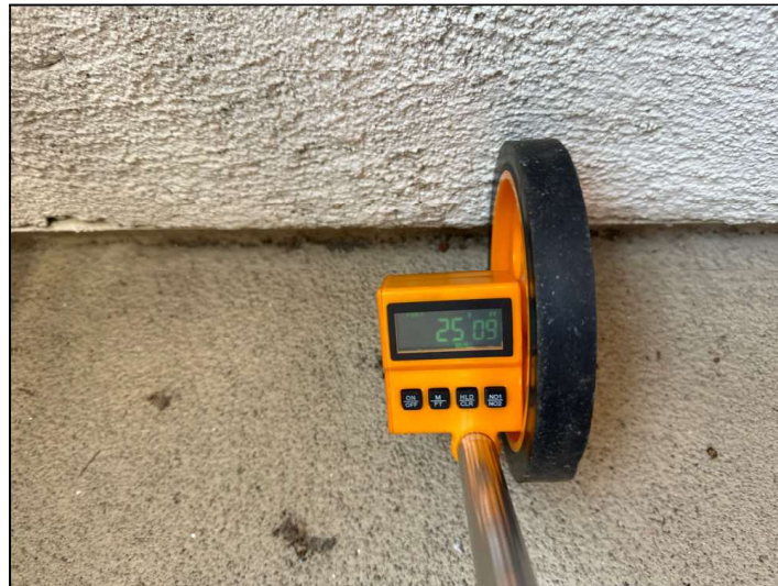
Measurement of balcony in one direction.
