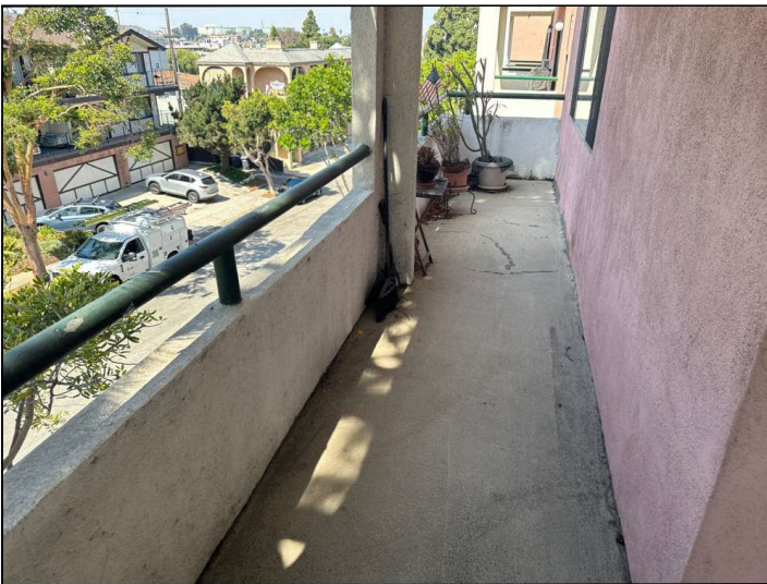
No visible structural problems were observed at the time of inspection.
