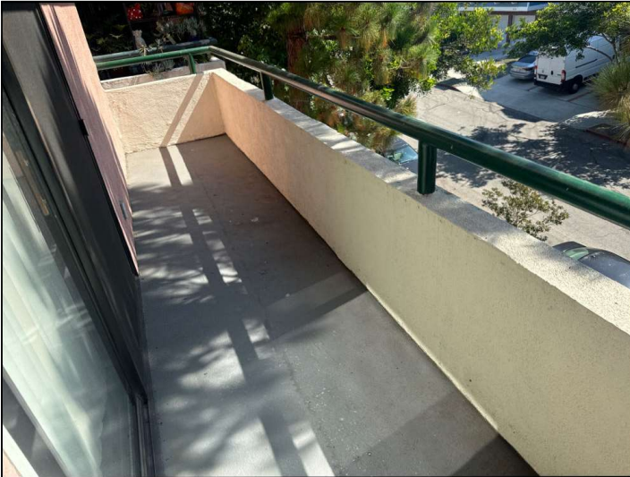
No visible structural problems were observed at the time of inspection.
