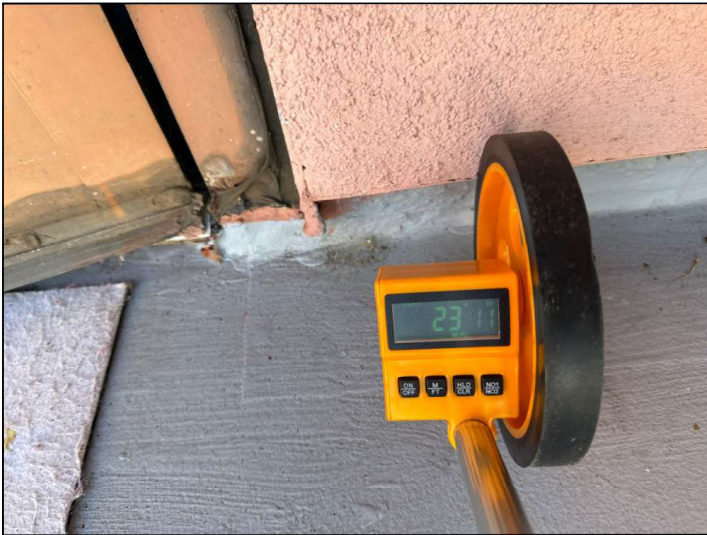
Measurement of balcony in one direction.
