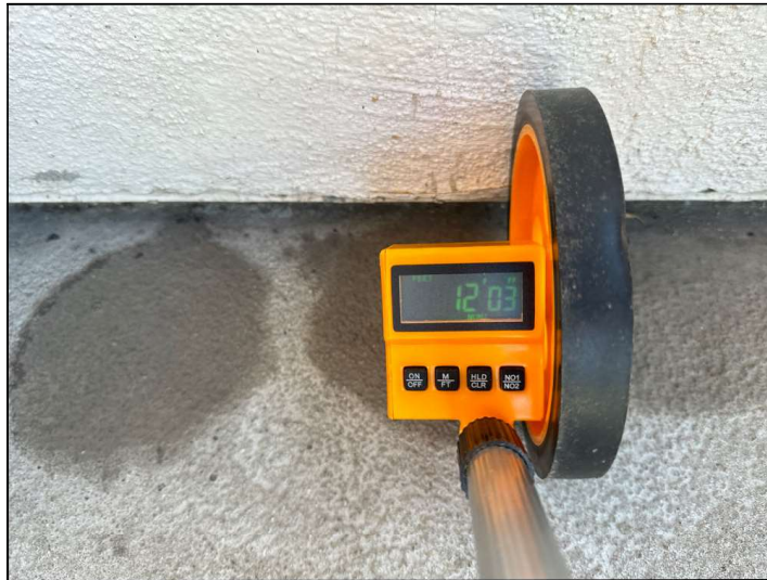
Measurement of balcony in one direction.
